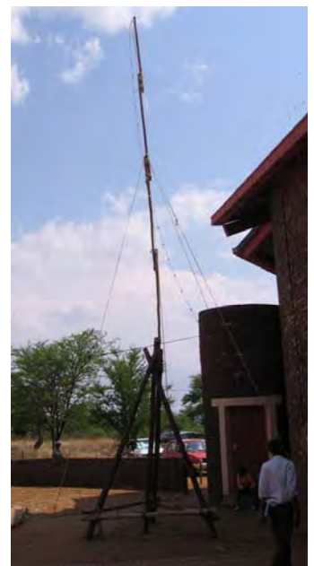
Our all-band, Scout-constructed vertical HF antenna.
